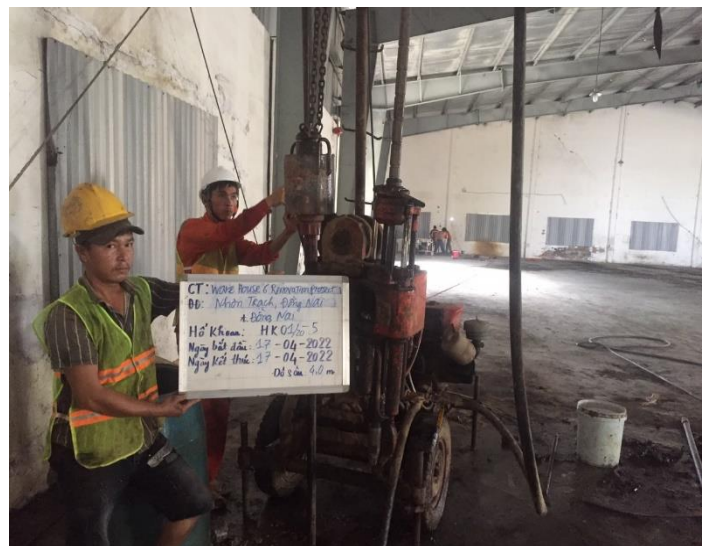
(Picture 1: Tone drill rig XY-100 )
